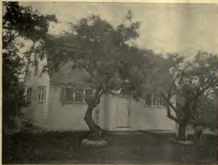
PUBLIC LIBRARY, LEVERETT, MASS. KARL S. PUTNAM, ARCHITECT. ERECTED 1916. COST $3500. CONTAINS ADULT READING ROOM, CHILDREN'S ROOM AND AN AUDITORIUM UNDER THE ROOF. THE LOT SLOPES AWAY AT THE REAR MAKING POSSIBLE A LIGHT, AIRY BASEMENT. OLD APPLE TREES ARE AN INVALUABLE DECORATIVE ASSET
