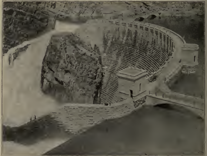
The water in the big pond made by the Roosevelt Dam would bury the whole State of Delaware a foot deep. Named after President Roosevelt, the dam was formally opened by him March 18, 1921. It is curved upstream so as to offer the resistance of an arch to the tremendous pressure of the water. (Pictures reduced in size.)
