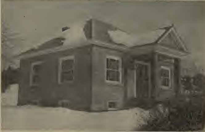
A LIBRARY DESIGNED AND BUILT BY A LOCAL CONTRACTOR IN 1921. COST $4750. CONCRETE BLOCKS AND METAL CEILING AND WALL COVERING USED TO SAVE MONEY AT THE
