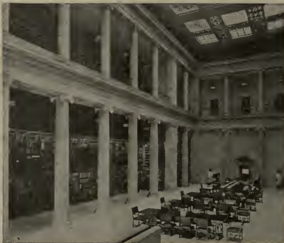
READING ROOM IN THE HILL LIBRARY
