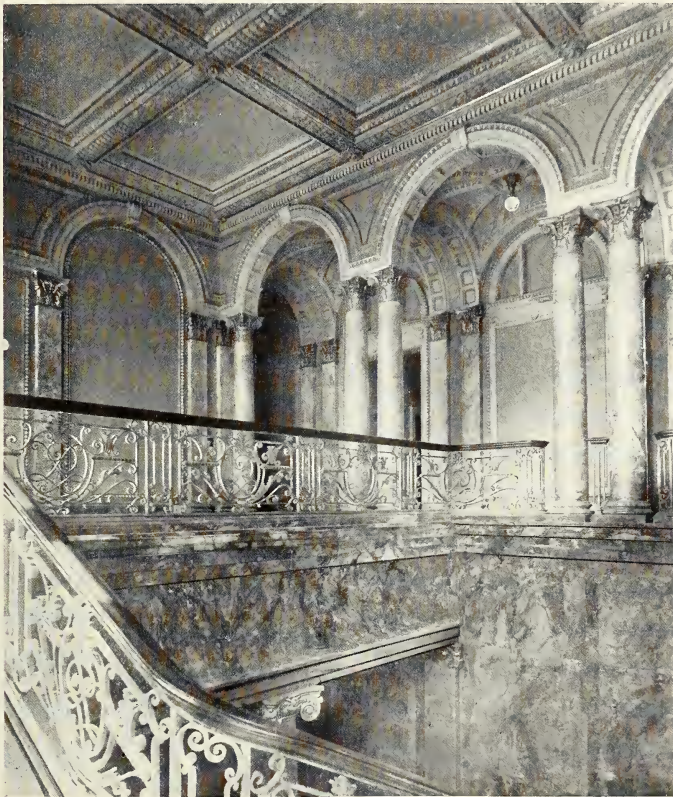
STAIRWAY AND CORRIDOR, PROVIDENCE LIBRARY.
