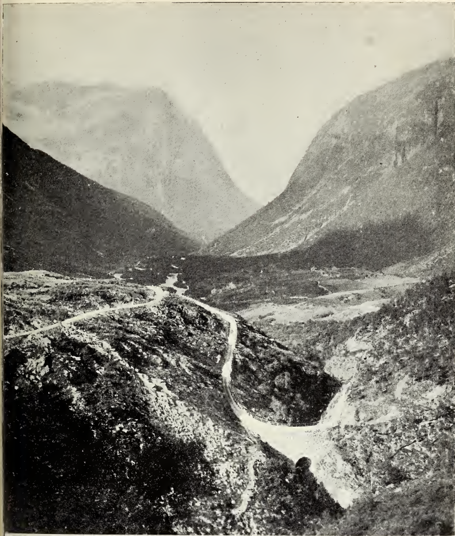
BRIDGES BOTH STRAIGHT AND CURVED.
