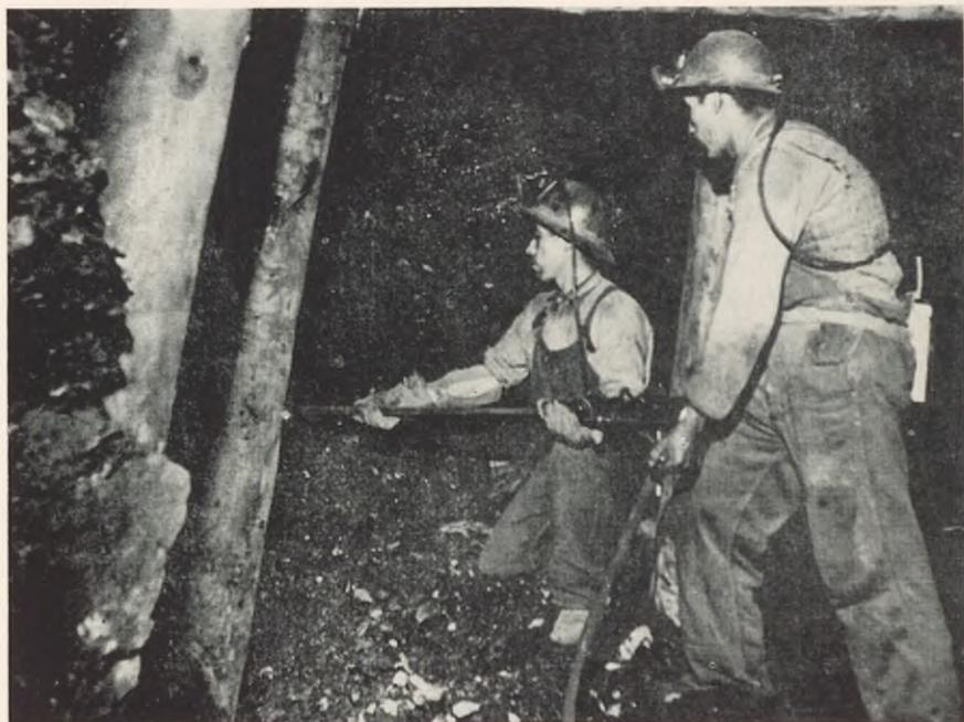
*Dry drilling in a coal mine*
