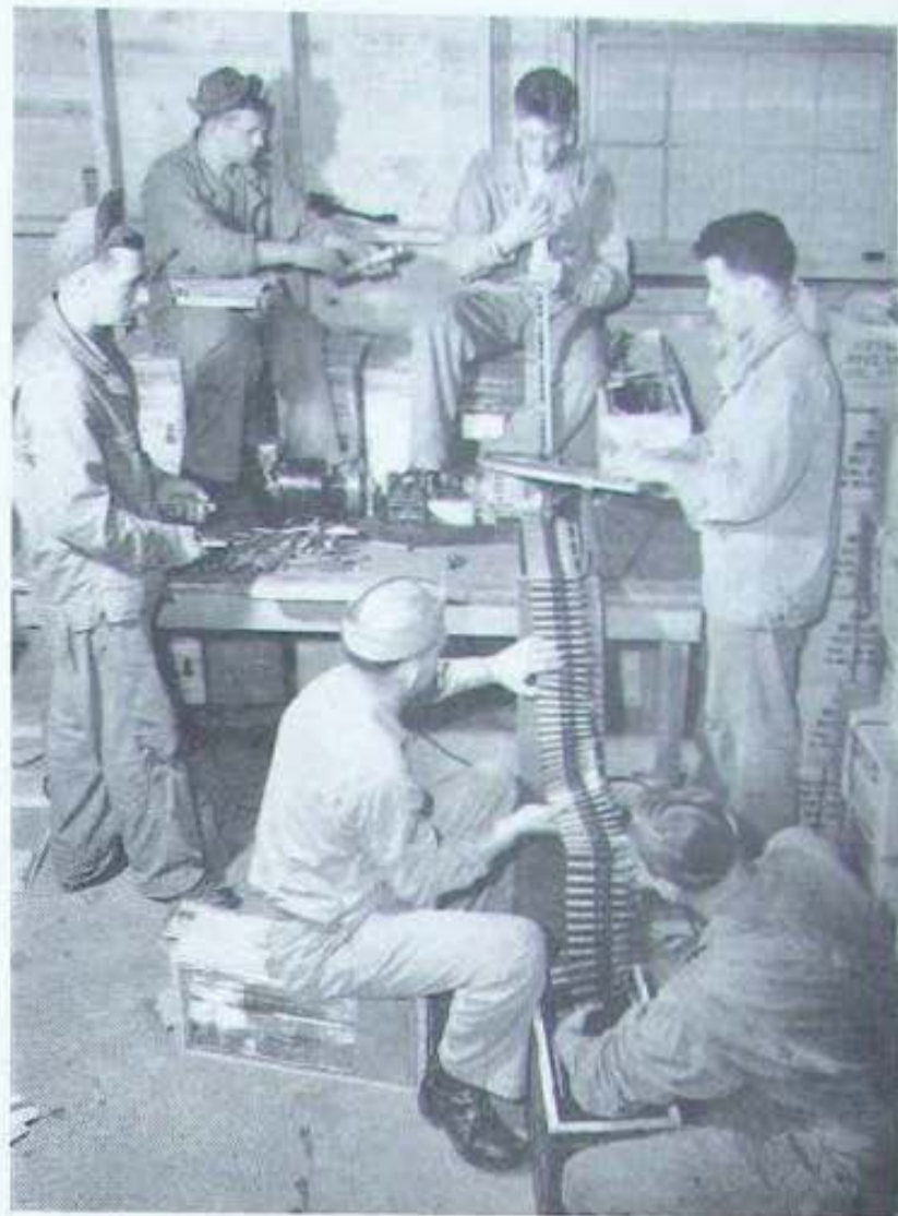
Belting fifty caliber armor piercing and tracer ammunition on automatic belting machine.
