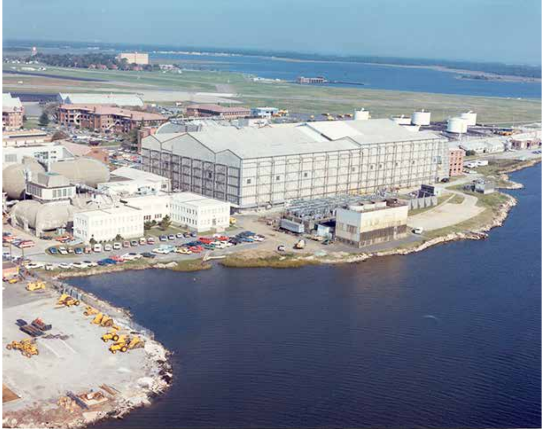
The huge Langley Full-Scale Tunnel building dominated the skyline of Langley Air Force Base for 81 years (1930–2011). The results of critical tests conducted within its massive test section contributed to many of the Nation's most important aeronautics and space programs. (NASA L-79-7344)
