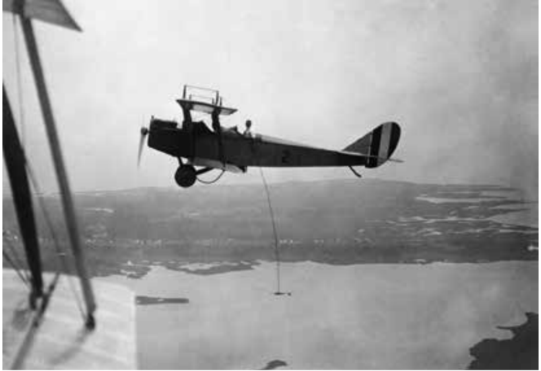
The National Advisory Committee for Aeronautics (NACA) began flight research projects at Langley Field in 1919 using airplanes borrowed from the military. A Curtiss JNS-1 "Jenny" is shown in flight with a trailing pitot-static tube for airspeed calibration in August 1922. (NASA EL-2001-00375)
