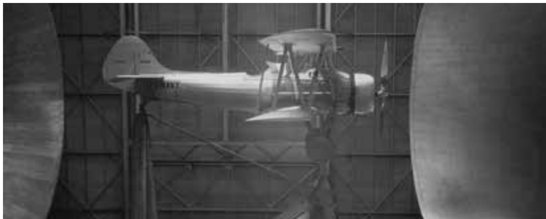
Tests of the Vought XO4U-2 biplane in the Full-Scale Tunnel in April 1933 were designed to investigate cooling characteristics of two-row radial engines. (NACA 8501)
