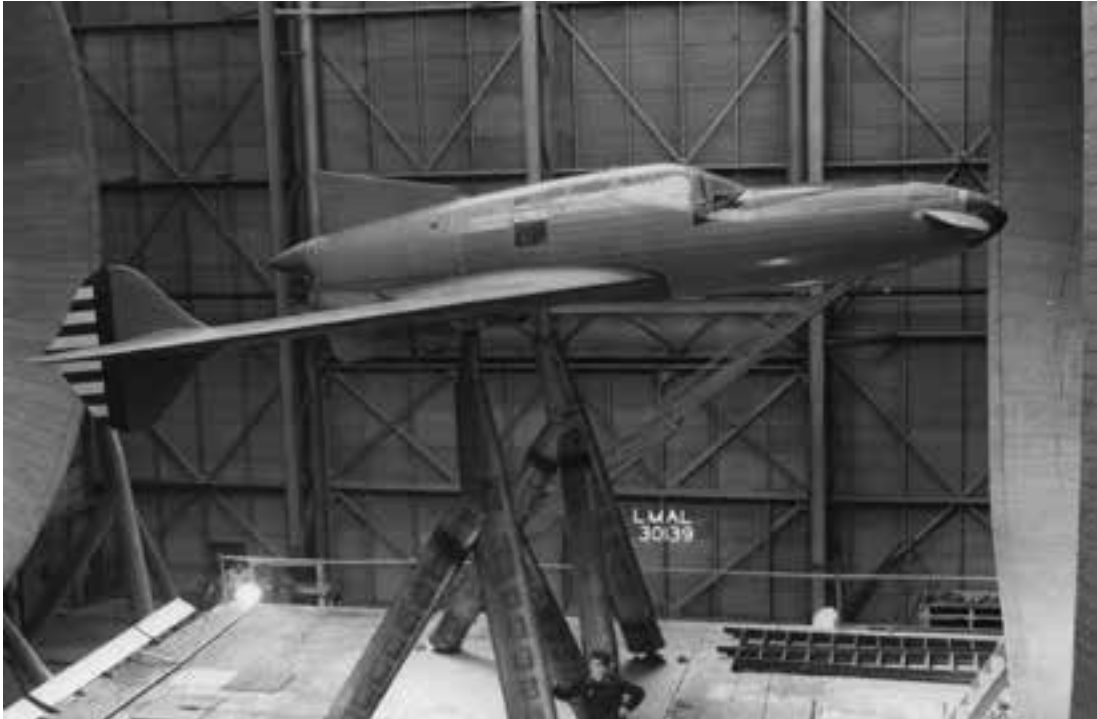
The radical canard-pusher Curtiss-Wright CW-24B flying demonstrator was tested in October 1942. Note the free-floating canard surface at the nose of the aircraft. The CW-24B was one of the first swept-wing aircraft. (NACA LMAL 30139)
