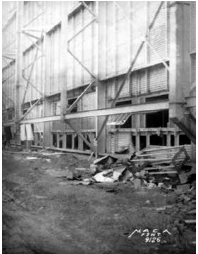
The 1933 hurricane caused widespread damage at Langley and the local areas. As shown on the left, most of Langley Field was flooded with several feet of water. Damage to the Careystone sheeting and windows of the Full-Scale Tunnel (above) was extensive, as water flooded the office and test section areas. (U.S. Air Force and NACA 9126)
