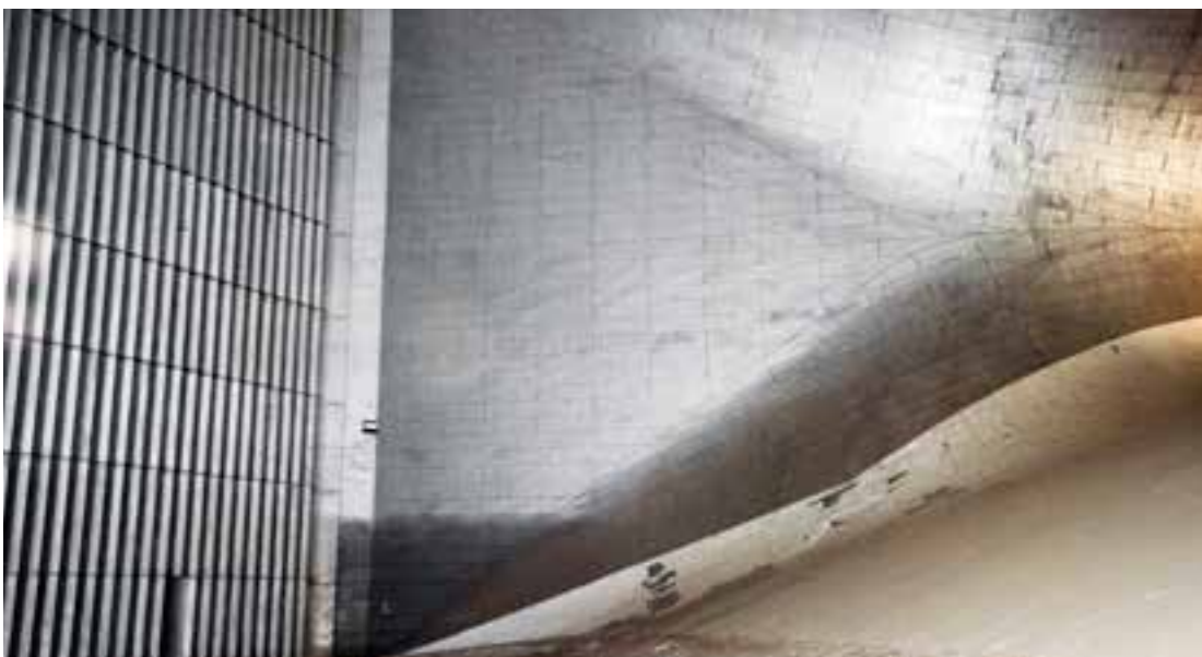
Photograph of the east side of the entrance cone shows details of the modifications to the corners installed following the unacceptable first tests in 1931. (NASA 2011-L-00037)
