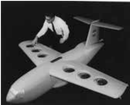
Project engineer Bill Newsom poses with a generic model of a lift-fan transport configuration that was tested with a variety of lift-fan arrangements. (NASA L-67-7754, L-67-7849, and L-67-7850)
