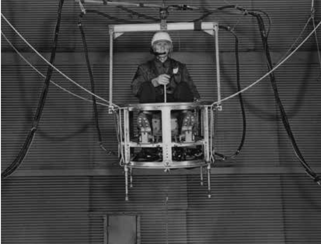
Langley test pilot Bob Champine flies the "flying chair" apparatus during proof-of-concept testing to develop the servomechanism concept required for the development of the famous Langley Landing Research Facility. The evaluation was conducted in a return passage of the Full-Scale Tunnel in 1962. (NASA L-62-1458)
