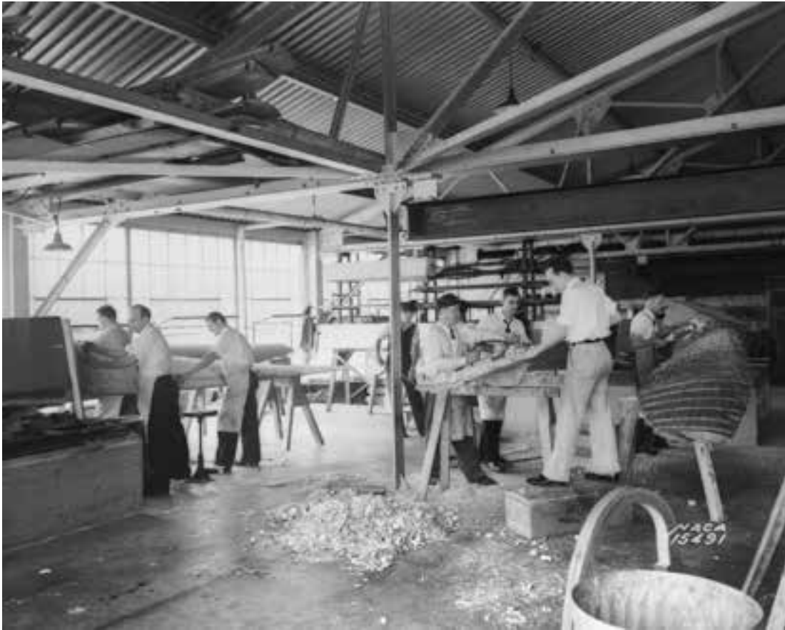
Langley woodworkers fabricate new wooden blades for the Full-Scale Tunnel in the flight hangar in May 1938. Made of Sitka spruce, the blades were installed a few months later and remained operational through the life of the tunnel. (NASA EL-2000-00357)
