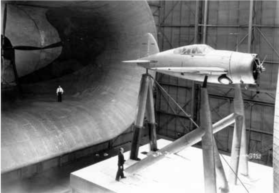
An urgent Navy request to examine the possibilities for increasing the top speed of the Brewster Buffalo in 1938 resulted in a parade of prototype and production military aircraft to the Full-Scale Tunnel for drag cleanup. This test was the last to use the tunnel's metal propeller blades before the change to wooden blades. (NACA 15336)
