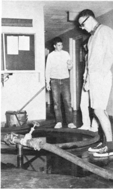
Filling the moat from the Alley 2 head.
