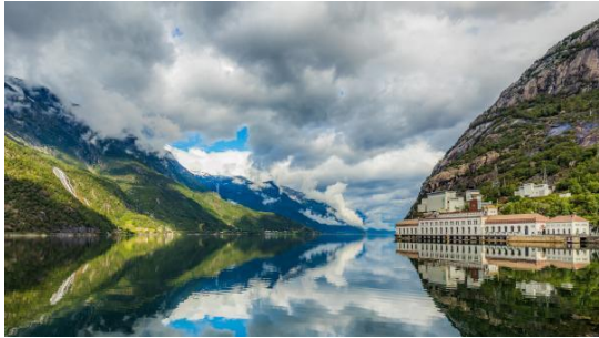
This photo of Tyssedal hydroelectric plant won the Norwegian first prize. Three of the photographer's images came in at top ten. Photo: Jorulf Kyrkjeide. CC BY-SA 4.0.
