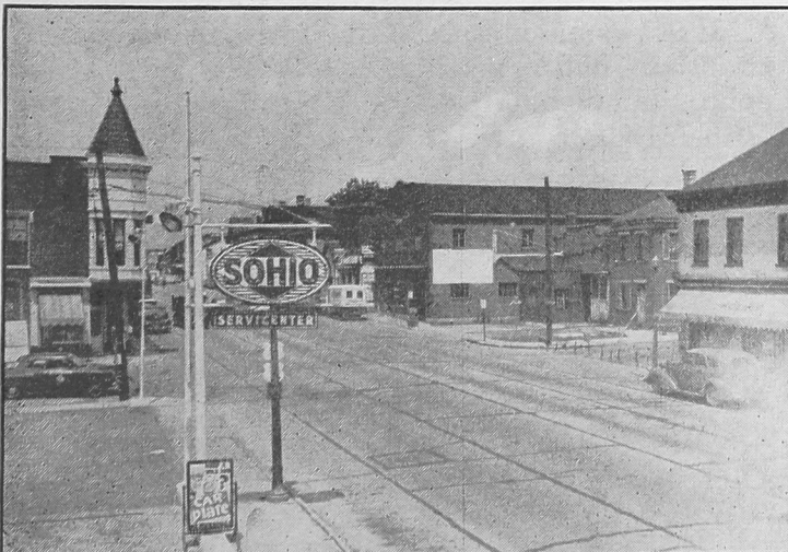
BENSON & READING RD. LOOKING NORTH—1951
