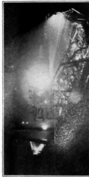
Lighting arrangement for pouring concrete at night, at abutment Pier 19. November 6, 1922.
