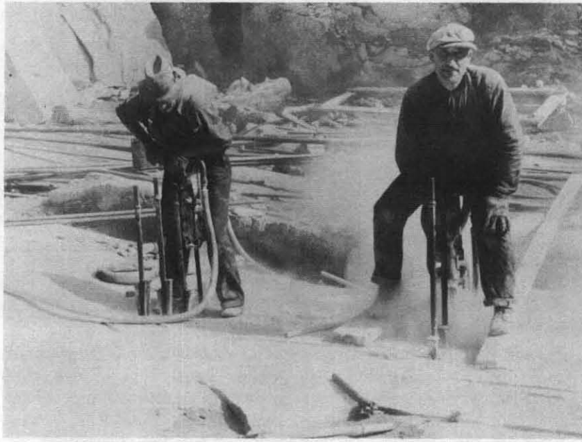
FIGURE 12. Jackhammer drilling without dust control. (About 1936.)
