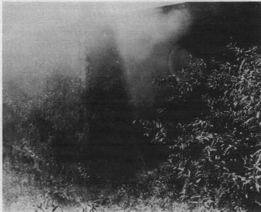
FIGURE 3. Attempts at controlling dust in granite sheds consisted of exhaust fans located in windows or openings in the sheds. Picture shows exhaust from sandblast discharging dust into outside air. Dust exhausted in this way could easily reenter the shed. (About 1925.)
