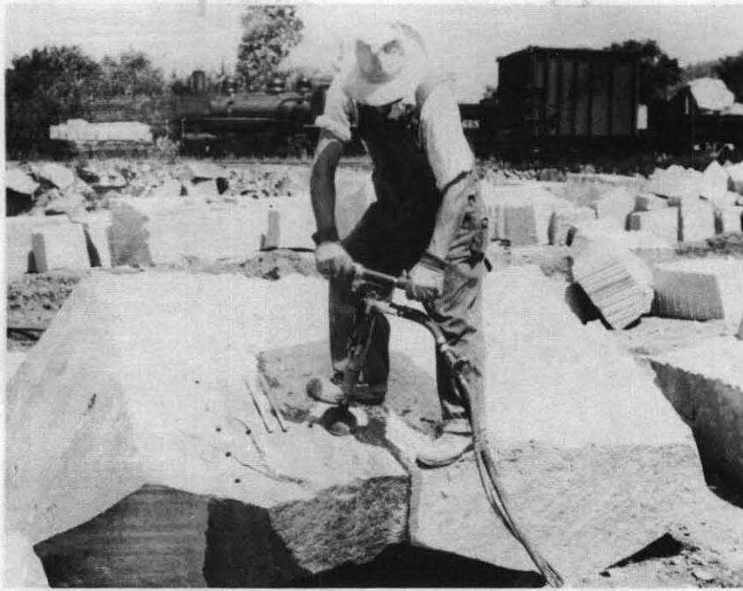
FIGURE 8. Modern wet drilling with jackhammer in plug yard. Rubber cup prevents spraying operator with water. (Courtesy of Rock of Ages.)
