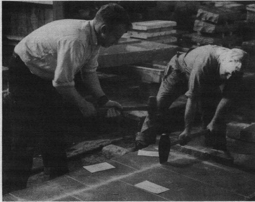
FIGURE 25. Breaking slabs with sledge and bull set. (1955.)
