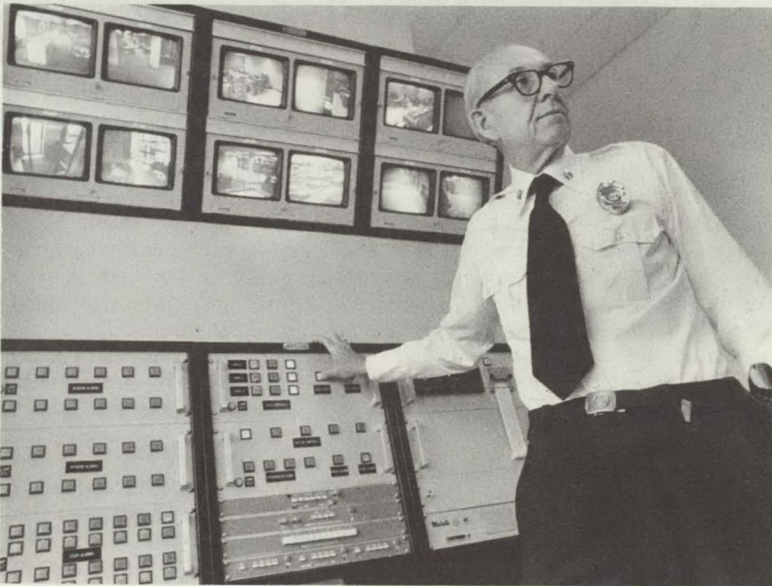
Security control module.
