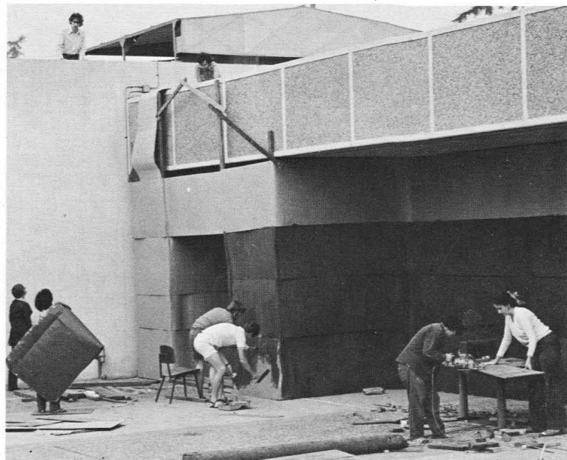
Repair work still under way.
