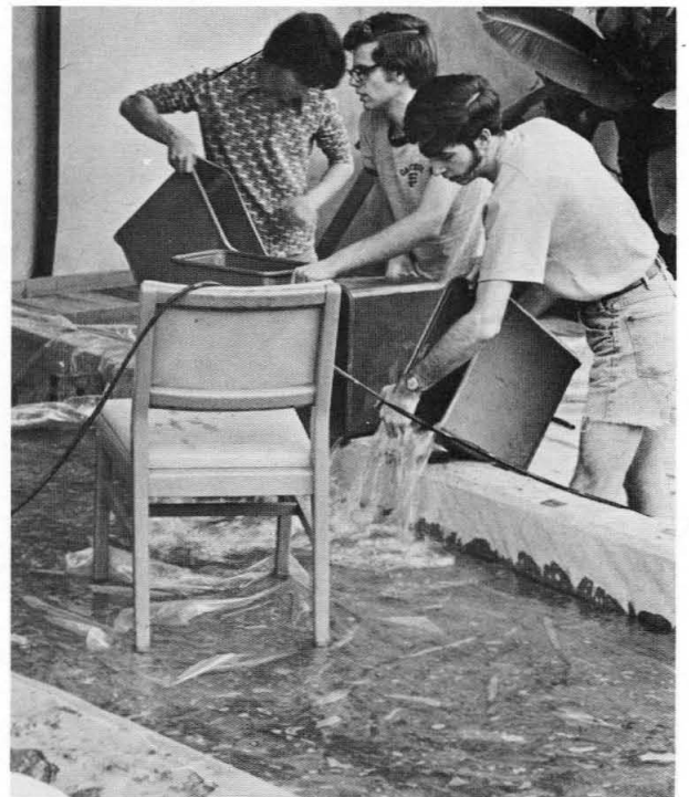
Repair work is proceeding well
