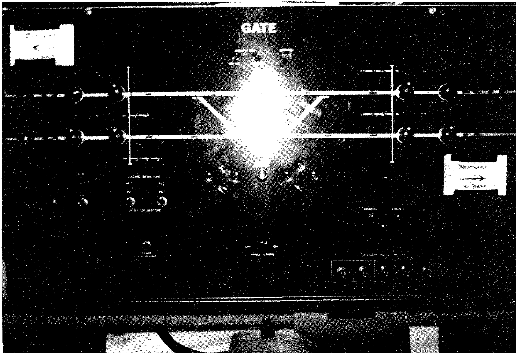
Figure 8.--Gate control panel. (Hand written labels not applied by the Safety Board.)
