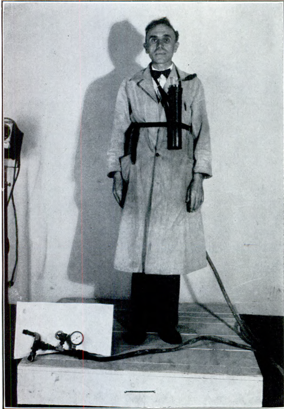
FIGURE 9.—IMPINGER SAMPLING TUBE ATTACHED ABOUT NECK OF WORKER.
