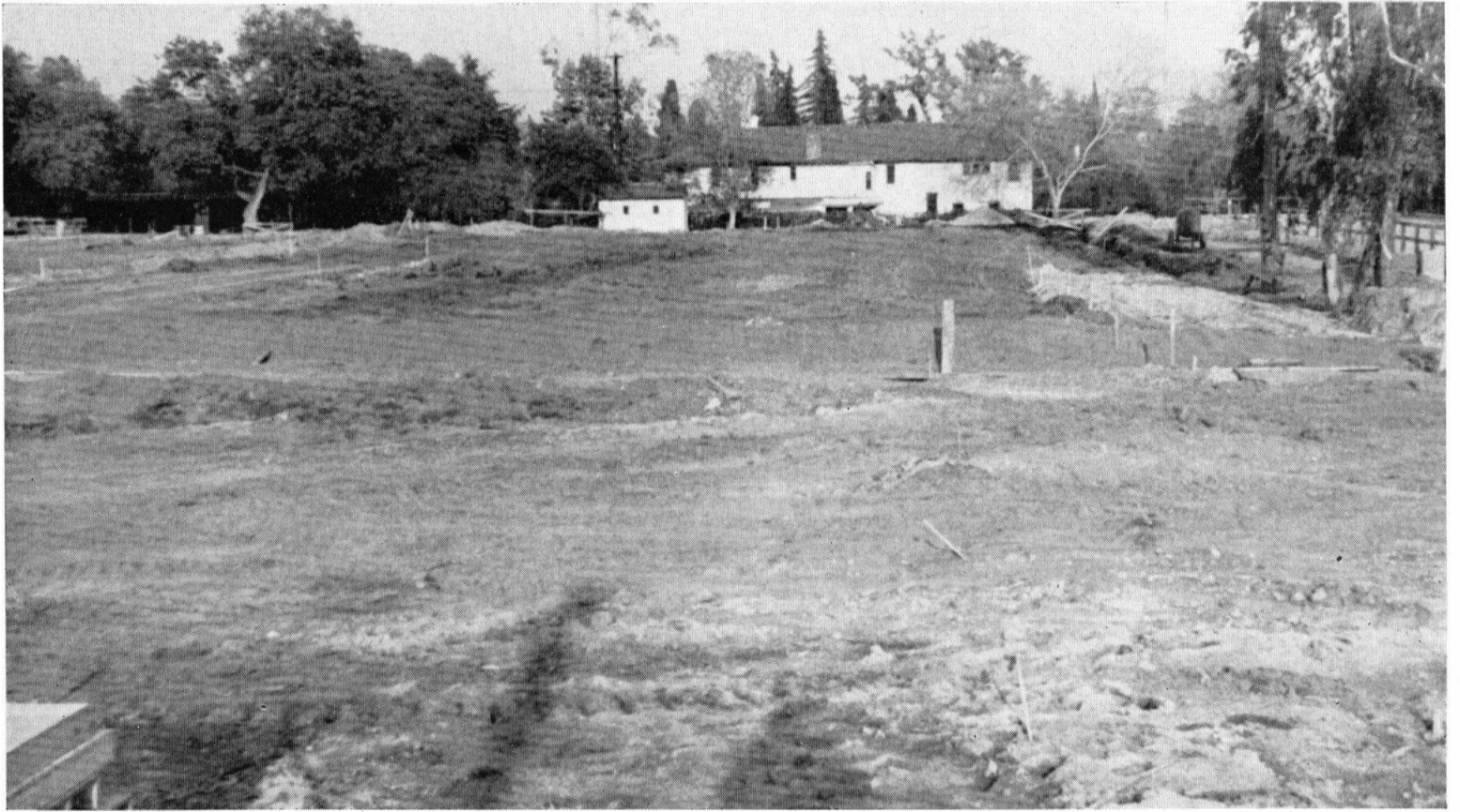
The Scott Brown Gymnasium and Alumni Swimming Pool under construction
